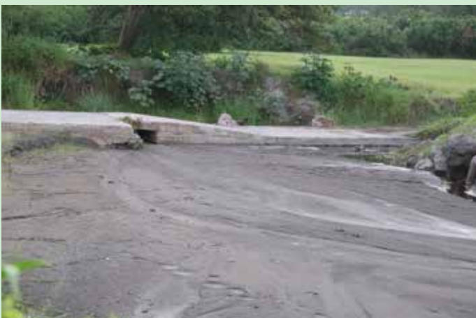
Below: The excavated old dock, now serving as a bridge over the link between the upper and lower parts of the Belham River Mouth.
